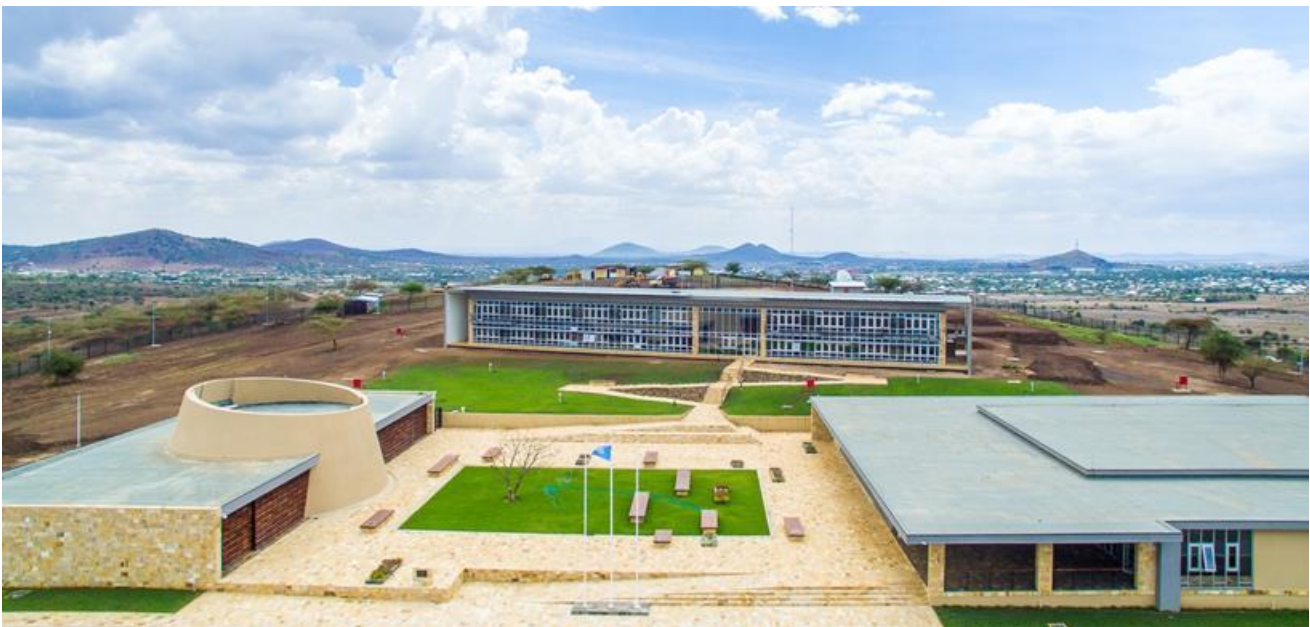
New Arusha premises of the Mechanism as at substantial completion, 1 December 2016
